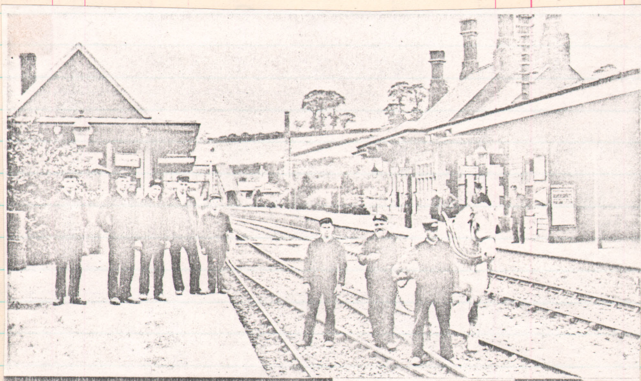
Crediton 1892. Ballasting over sleepers. (NRM Collection) 594/63
