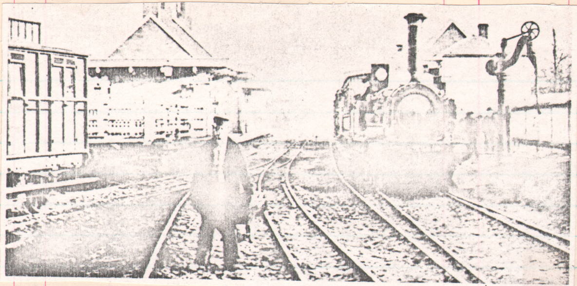
15962 LGRP Crediton 1880 Mixed gauges remaining after GWR (B&E) lease of N. Devon Railway. Broad gauge goods trains ran until 1892
