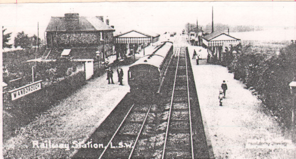
Wanborough (Guildford-Farnham). Bored sleepers (every 5th crib) possibly for track drainage to six feet.
