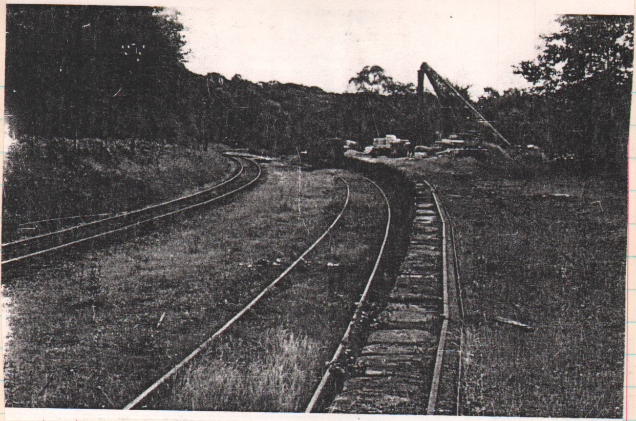
Biclade Wharf, Forest of Dean, 1947 Loading Bank
