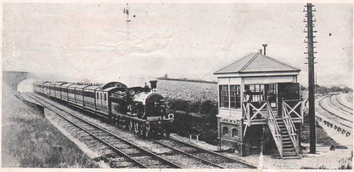
Winchester Junction c.1900. Fourth sleeper baring. Alton Line to right.
