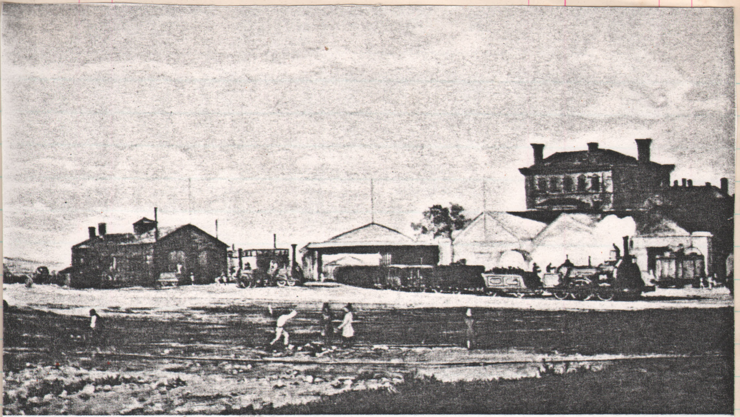
Southampton Terminus c. 1840. Work on track in foreground, (Original may show rails clearer - possibly chairs in places.)
