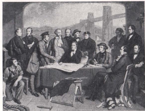
MENAI TUBULAR BRIDGE COUNCIL—ROBERT STEPHENSON PRESIDING.
