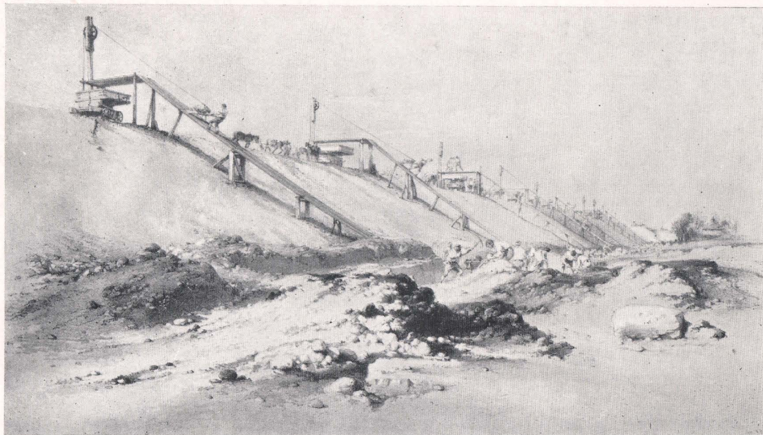
BOXMOOR EMBANKMENT, SHOWING METHOD OF EXCAVATION.
